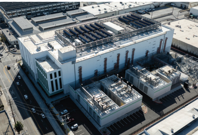
◀ Data center facility, Vernon, California.
